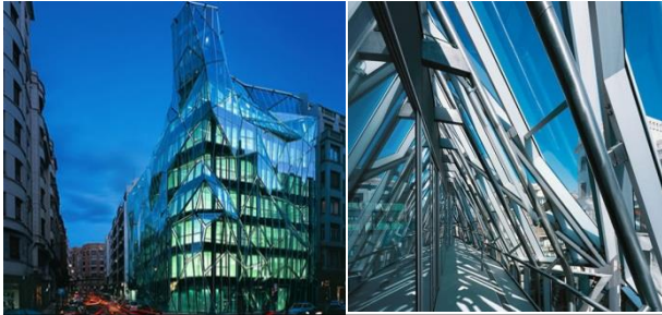
Figure 2: external folded double skin façade (left), social break out space in the cavity of the DSF (right)
