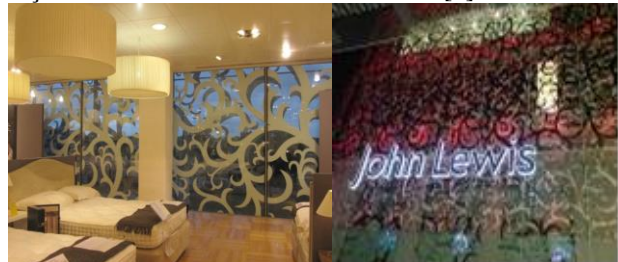
Figure 1: John Lewis Store in Leicester, 2008 by FOA where the external pattern is reflective and the internal pattern is matt etched on the glass. Both patterns directly face each other and this is to refract direct solar entry which is incident at an angle while allowing shoppers to
