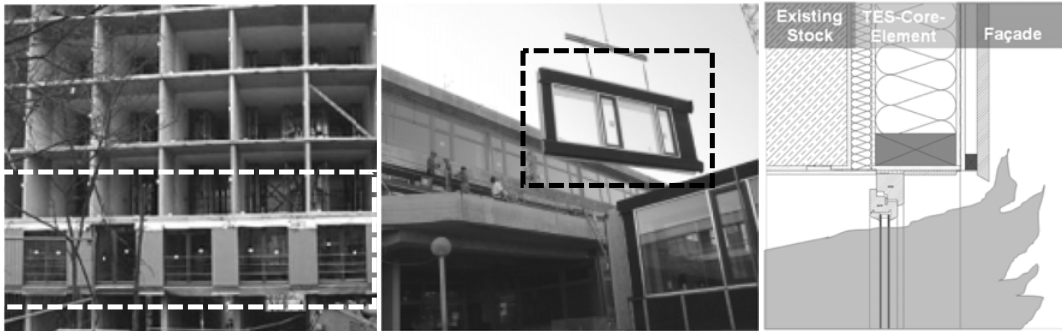
Figure 1. Mounting and Construction Section of a TES-façade.
