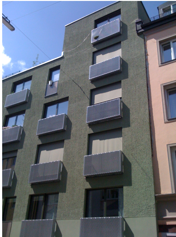
Figure 4.1: Southern façade of the multi-family house case study in the Schwanthalerhöhe neighborhood in Munich [146].
