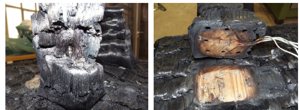
Figure 15: remaining cross section after 30 minutes fire test with insufficient wood coverage (connector type G)
