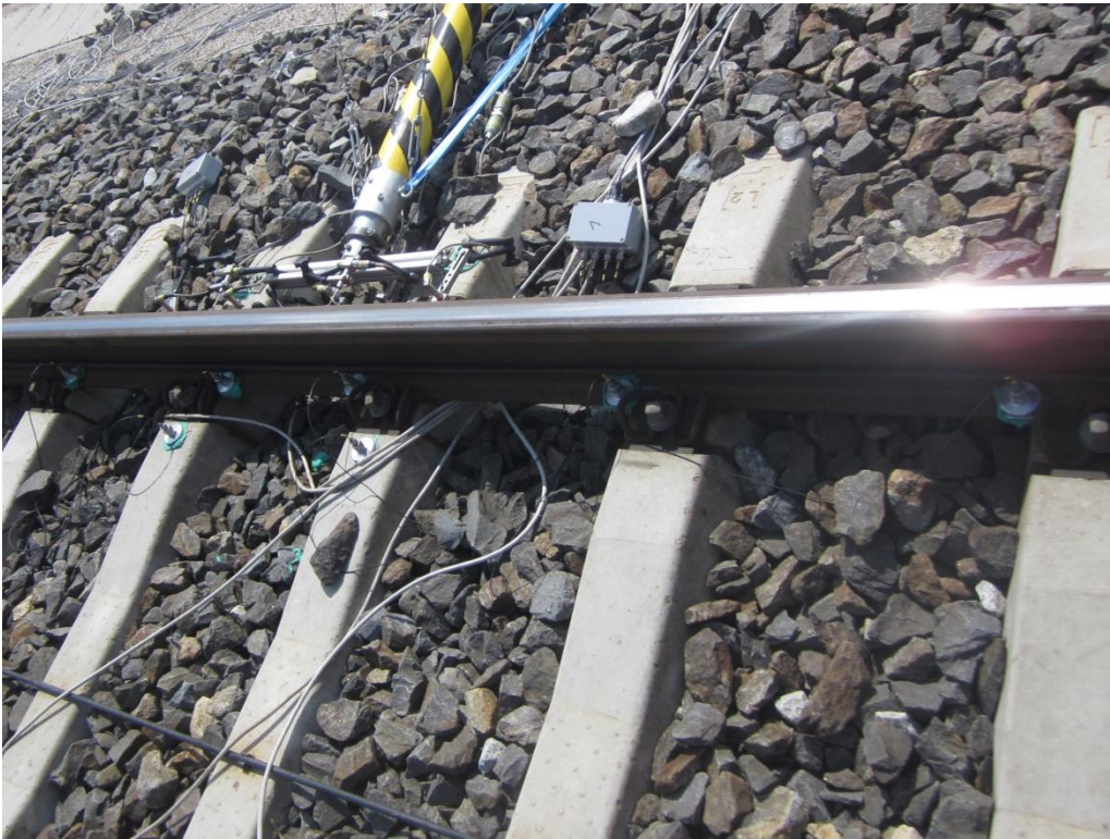
Pic 6: Installation of accelerometers
