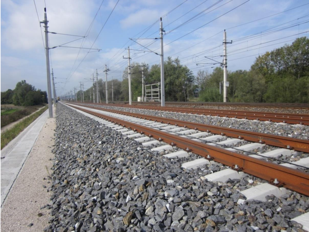
Pic 1: Overview of measurement section 3 (Ballasted track A-ÖBB)
