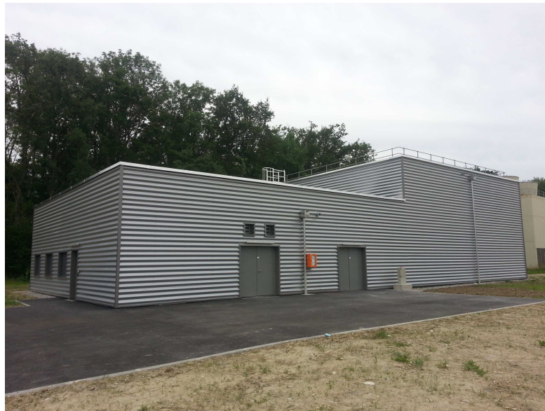
Figure 4.4: The RP calibration facility, building 772.
