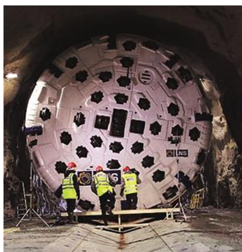
Fig. 45: Robbins open gripper TBM used at Røssåga tunnel (www-06).
