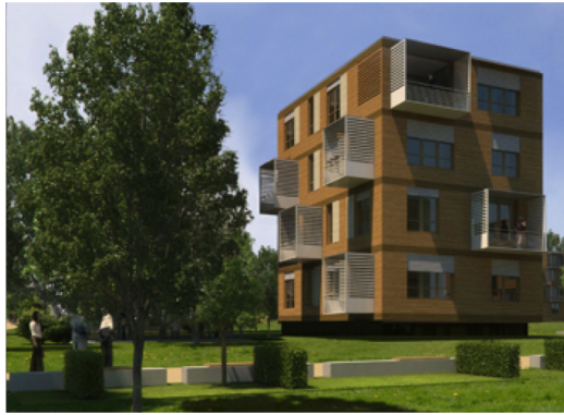
Figure 3.6: Four story timber building in Bad Aibling. [5]
