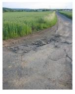
The width and the length of agricultural machines have extremely risen in the last years. Country lanes are still dimensioned on the size of the machines of 40 years ago. This can lead to problems especially in the curves.
