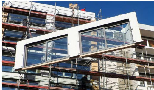
Figure 5: Mounting a TES-Element [gumpp&maier]
