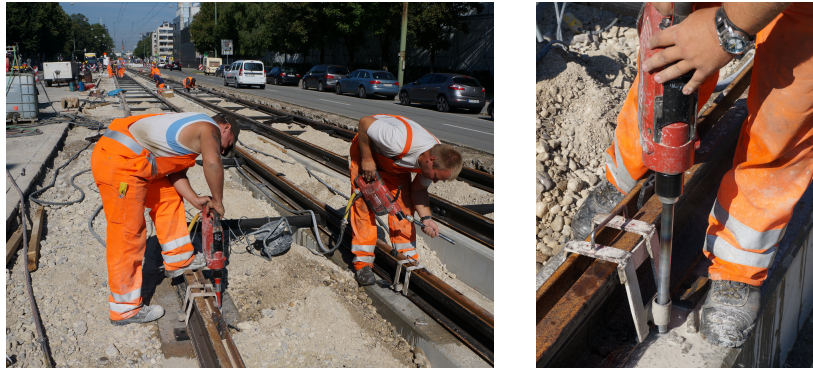
Drilling anchor holes to fasten tram rails using a drill template
