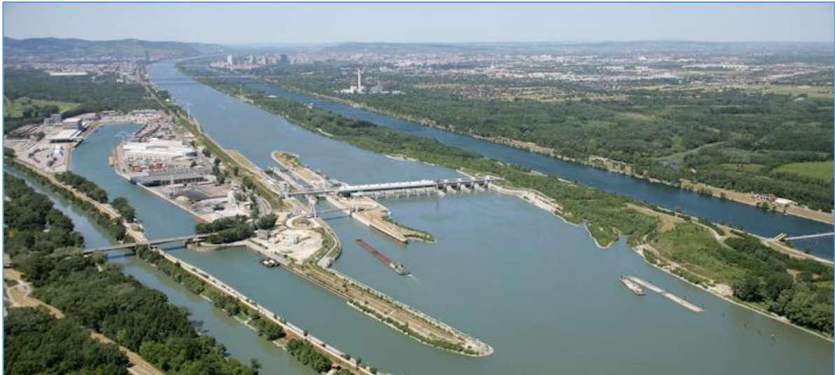
Figure 4.26 An aerial view of the Danube riverbed and the Danube Island (Vienna government, 2015)
