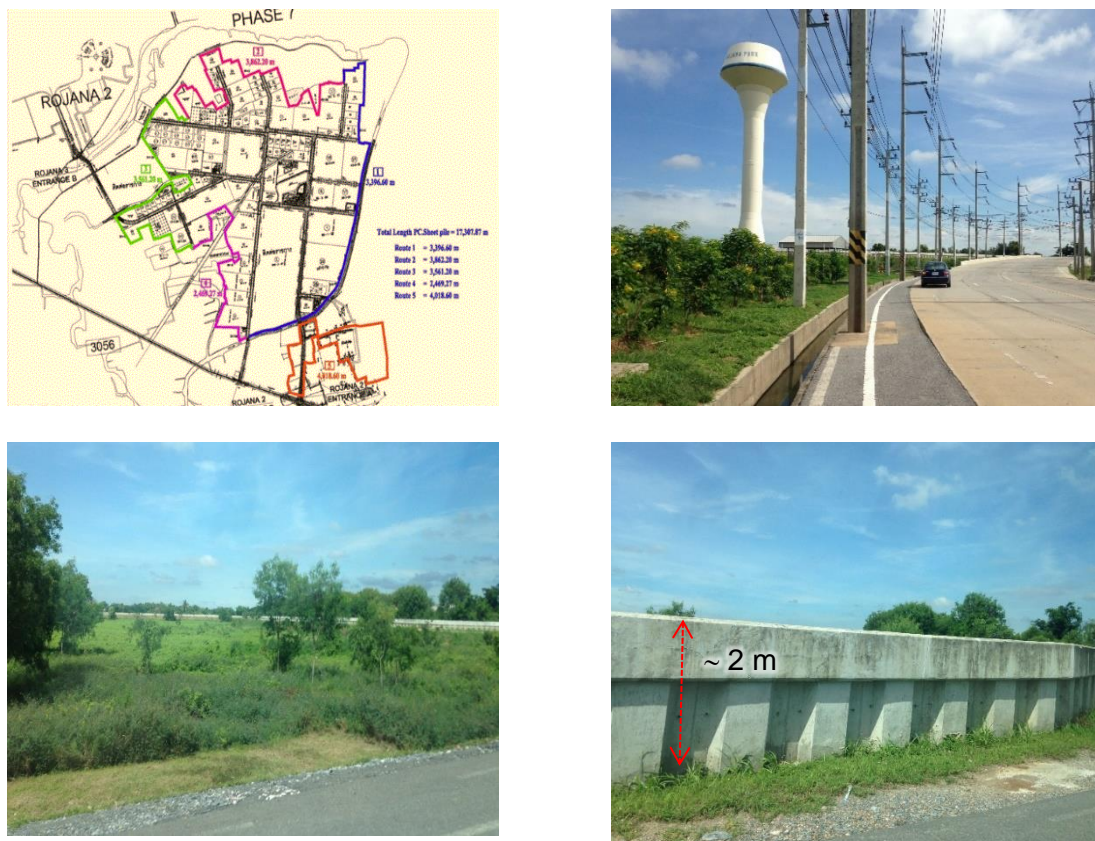
Figure 3.7 Private flood wall protection in Industrial Park, Ayutthaya province, Thailand (Author)
