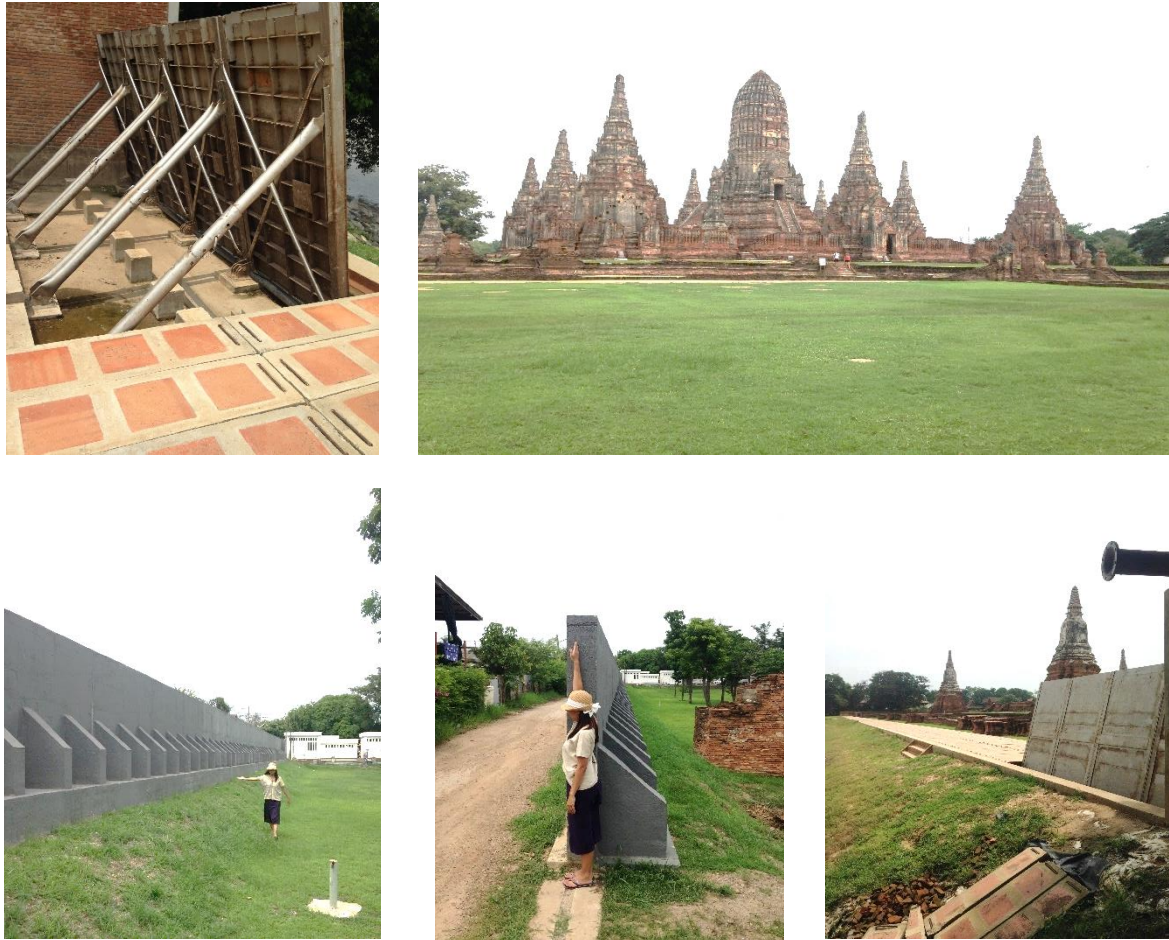
Figure 3.9 The public flood wall protection in Ayutthaya province 11 (Author)
