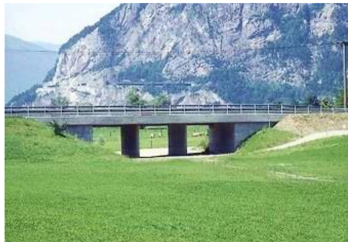
Figure 6.16 Highway A4 with room for the flood water to flow underneath (Fedier & Walker, 2008)
