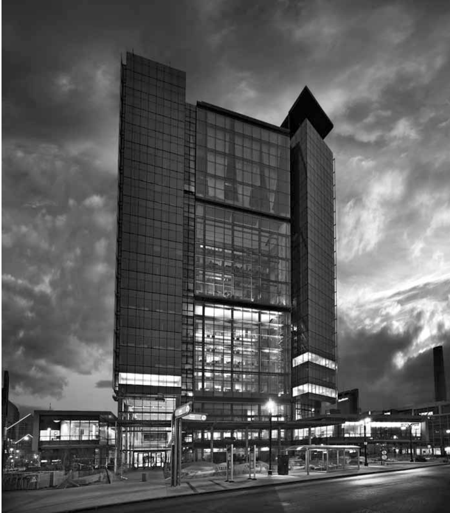
Manitoba Hydro Place designed by KPMB. Image courtesy of Gerry Kopelew.
