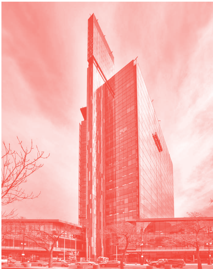
(above) Manitoba Hydro Place, Winnipeg, designed by KPMB.
