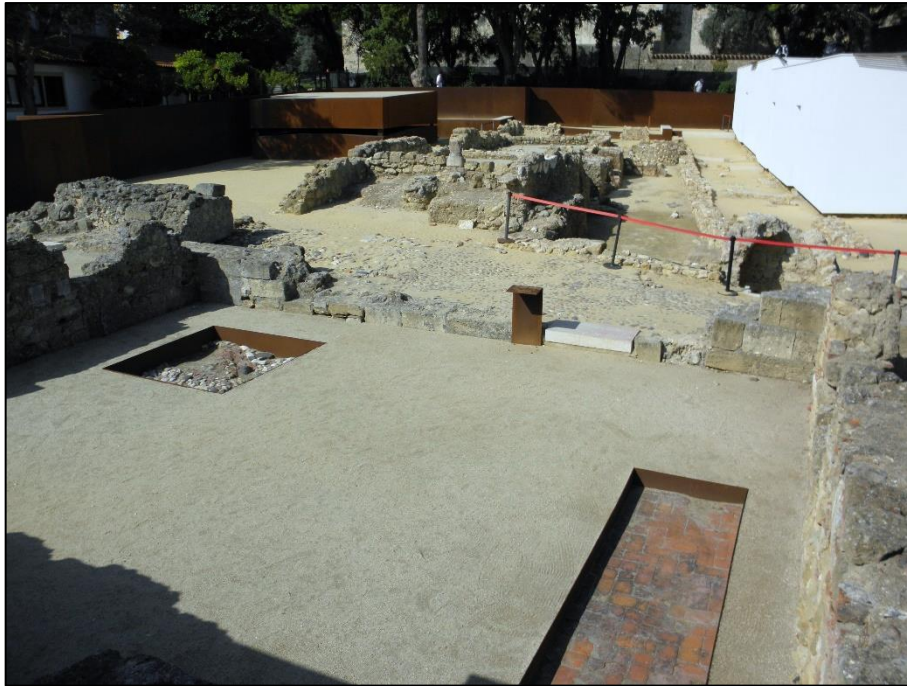
Fig. 20 Reburial of tile floor with exposed sections for monitoring at the Royal Palace of the Alcáçova, Lisbon, Portugal
