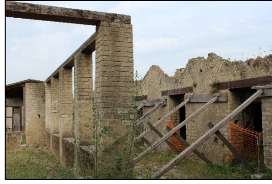
Fig. 2 (left) and 3 (right) Structural stabilisation preventing wall collapse at the World Heritage Sites of Pompeii (left) and at the Villa San Marco, Stabiae, Italy (right)
