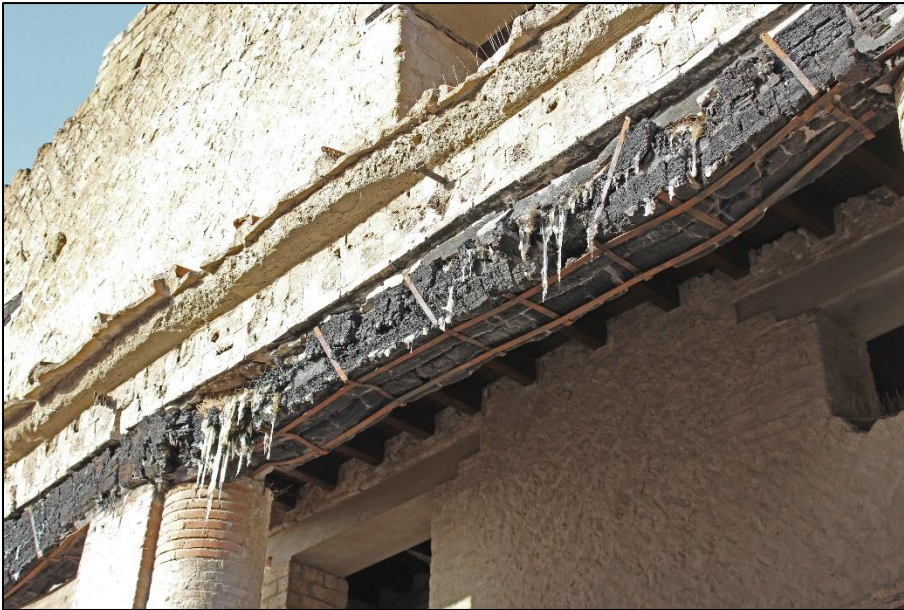
Fig. 18 Melting in the summer, wax used to consolidate original wooden lintel at the WHS of Herculaneum has created aesthetical and material reversibility problems
