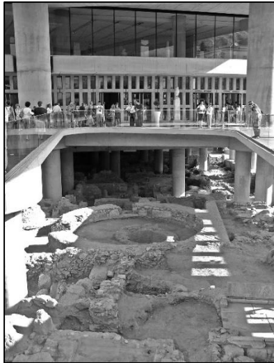
Fig. 13 (left) and 14 (right) The massive columns supporting the building of the New Acropolis Museum have been divided to three columns with smaller diameter to minimise damage to the remains of an ancient Athenian quarter
