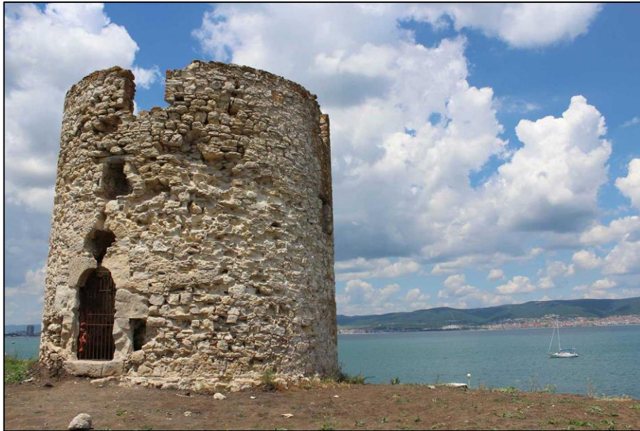
Fig. 51 Section of the fortified outer wall of the Ancient city of Nessebar
