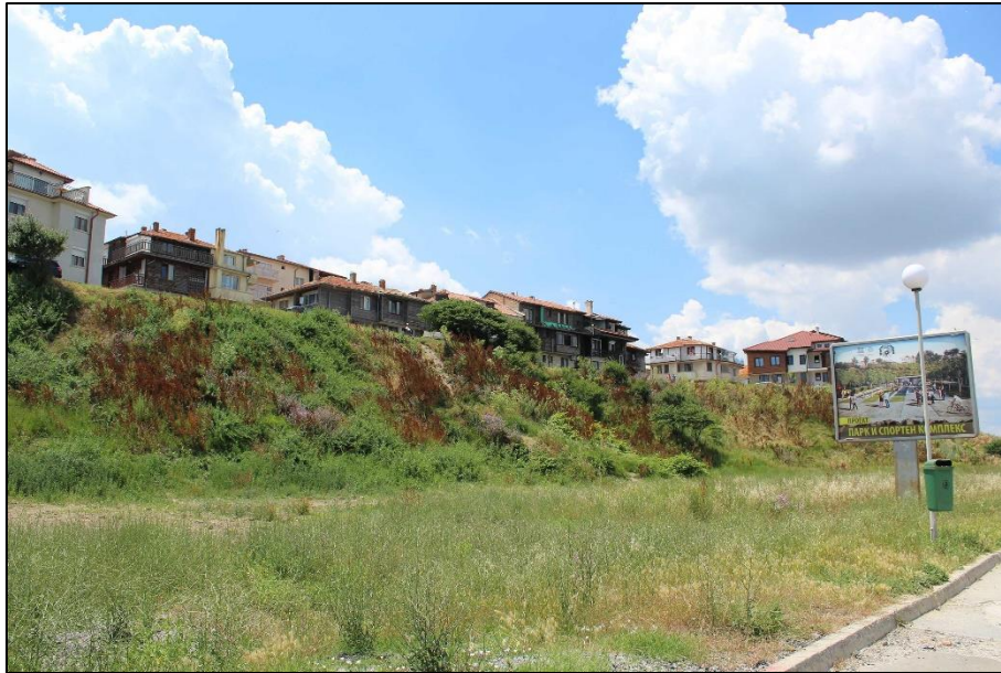
Fig. 61 The currently unused green area in the north part of the historic peninsula
