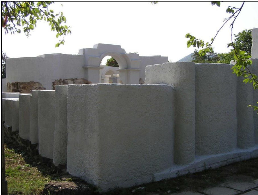
Fig. 33 Massive rebuilding of the Golden (Round) church at the archaeological site of Veliki Preslav, Bulgaria. Interventions of such type lack sensibility and completely obscure the survived original
