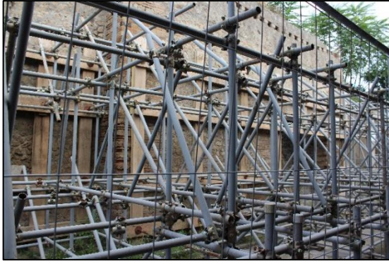
Fig. 2 (left) and 3 (right) Structural stabilisation preventing wall collapse at the World Heritage Sites of Pompeii (left) and at the Villa San Marco, Stabiae, Italy (right)
