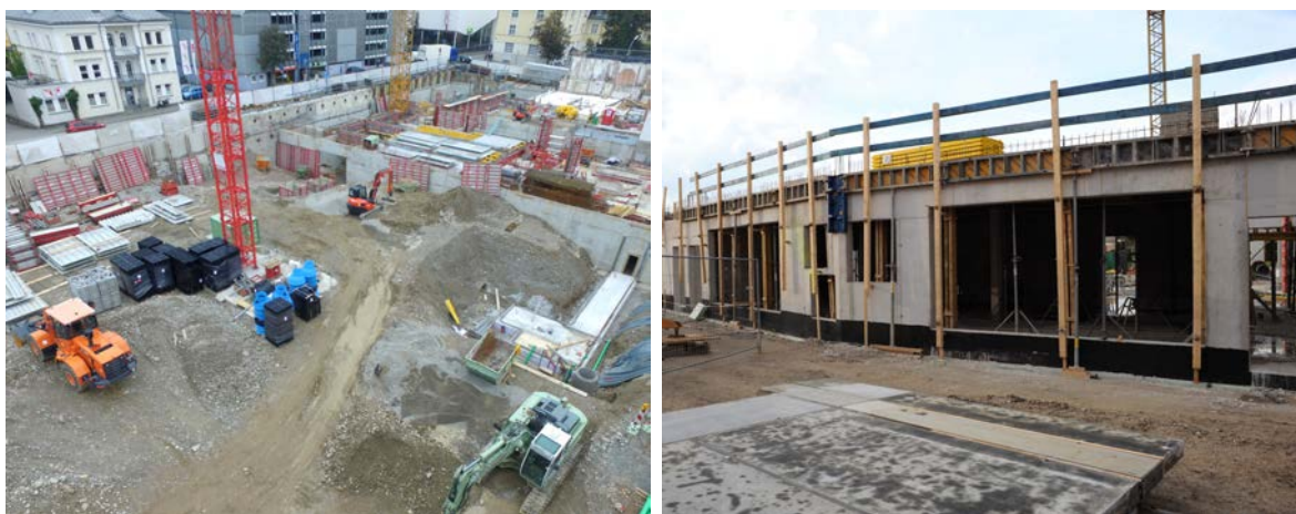
Figure 3.1: Aerial (left) and from ground taken (right) construction site photo
