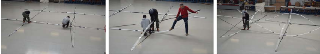
Figure 16: Assembly of the GRP-bundles
