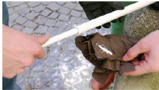
Figure 13: Gluing the GRP slot joints
