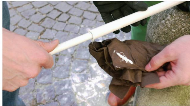
Figure 9: Gluing the GRP slot joints
