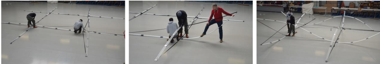
Figure 12: Assembly of the GRP bundles
