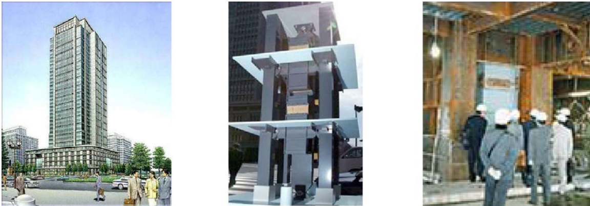
Figure 05: In 2002, “Shimbashira-Seishin” (Center Column Vibration Control) was applied to the 198 meter Marunouchi building in Tokyo. Left: View of the building Middle: “Shimbashira” as a major element of the structure Right: Connection between the “shimbashira” and the steel structure of the building.
