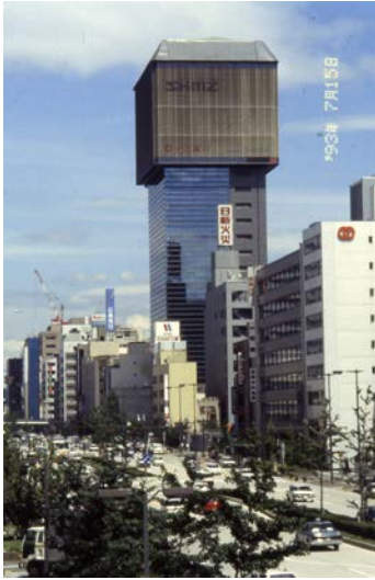
Figure 1: Shimizu's horizontally moving "Smart" factory in operation
