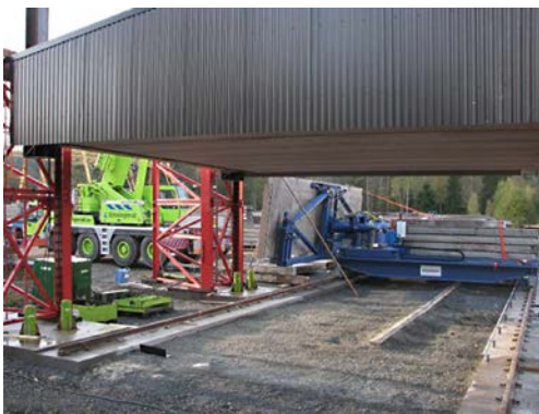
Figure 2: Skanska's prototype of an automated building construction system
