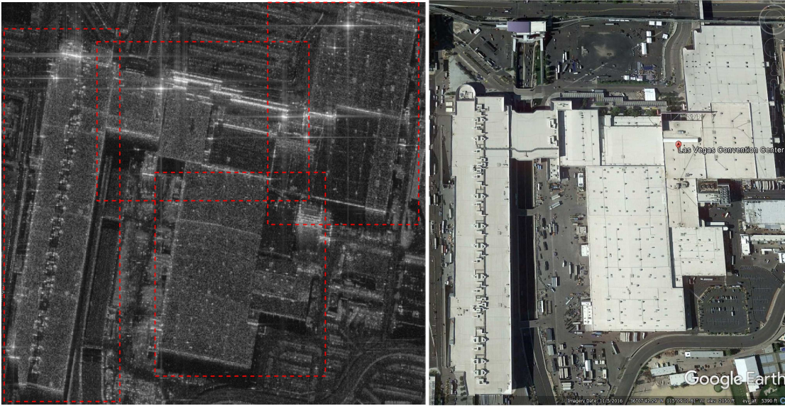
Figure 5.19: (Left) The TerraSAR-X test image of the Las Vegas convention center. Since the building structure is complex and its spatial area is large ( 800 \times 850 pixels), the four parts of the whole InSAR phase stack as cropped with the red dashed rectangles in the figure are separately processed. (Right) The associated optical image from Google Earth.
