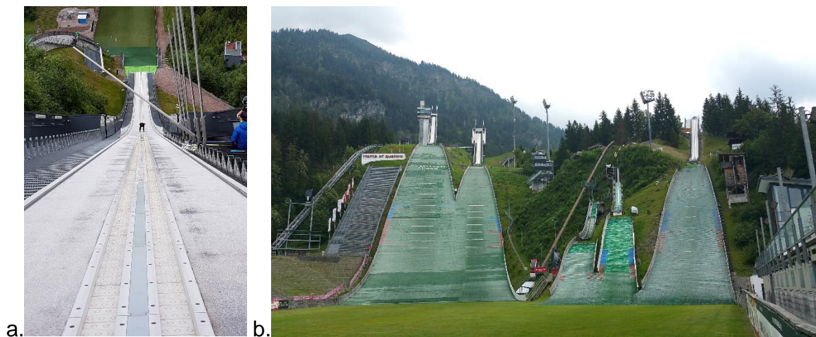
Figure 13. SkiJ hills during summer conditions. In-run of the HS100 in Oberhof (GER) where are notable the ceramic tracks in which water is flowing (a.). Landing area of the SkiJ hills of the Audi Arena in Oberstdorf (GER). The hill used in the study is the second from the left (HS106) (b.).
