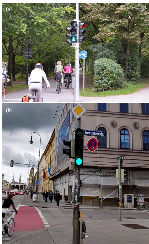
Figure 2. Installed countdown timer displays in Munich at (a) the crossing “Milbertshofener Straße / Christoph-von-Gluck-Platz” (permanently installed), and, (b) the intersection “Ludwigstraße / Theresienstraße” (installed for one day).
