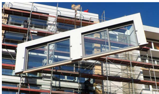
Figure 5: Mounting a TES-Element [gumpp&maier]
