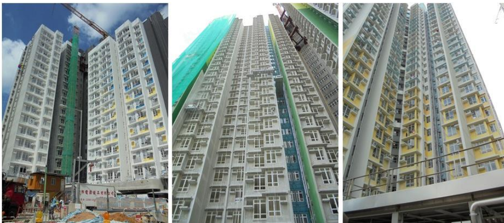
Figure 42: The typical types of public housing façade design in Hong Kong, source: (Wen Pan).
