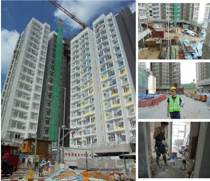
Figure 26: Snapshots of the on-site visit, and the case study building.
