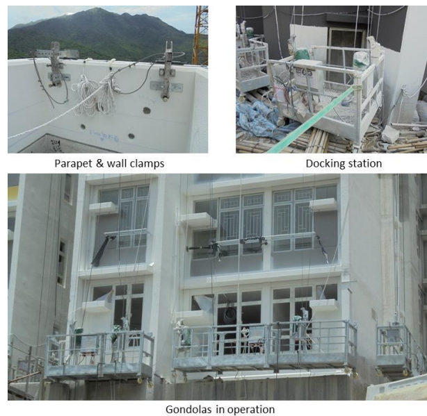
Figure 37: Gondola components and installation.
