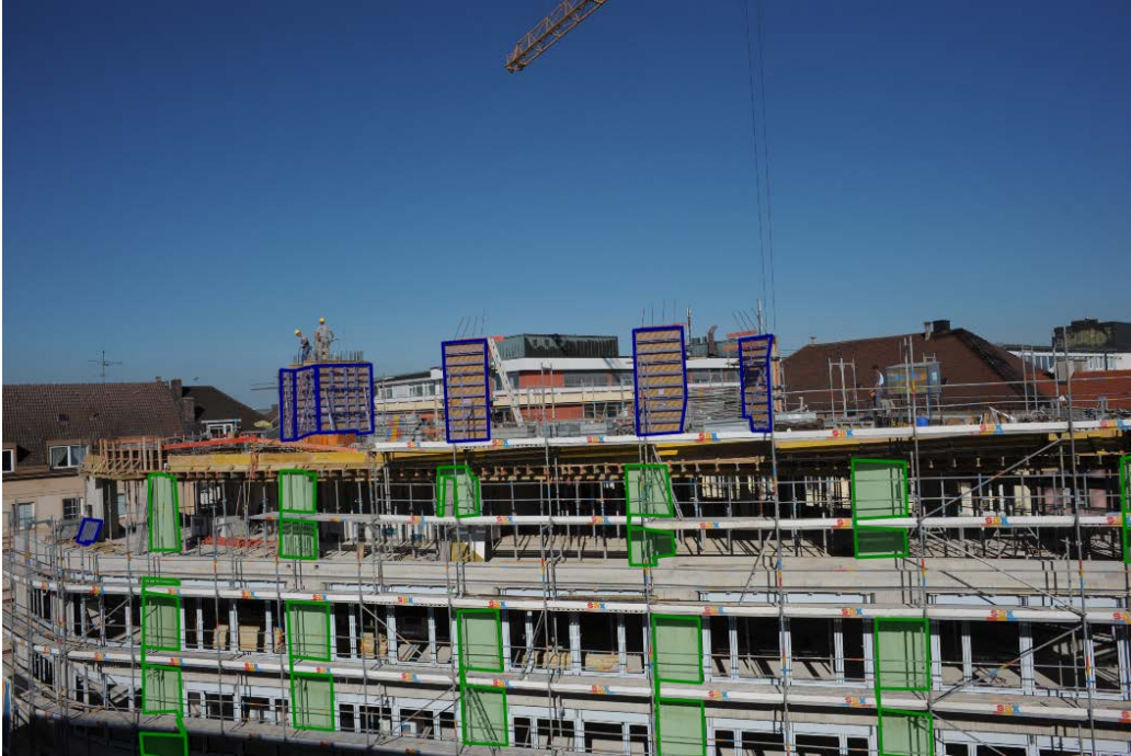
Figure 6: Sample image of the labeling process. Displayed are the labeled formwork (blue) and column (green) elements. During this research, Labelbox [47] is used for labeling.
