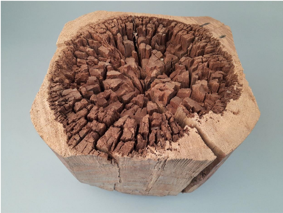
Figure 5 Brown rotted wood, showing the typical brown colour and the cubic cracks. Image: M. Risse, Holzforschung München, TUM
