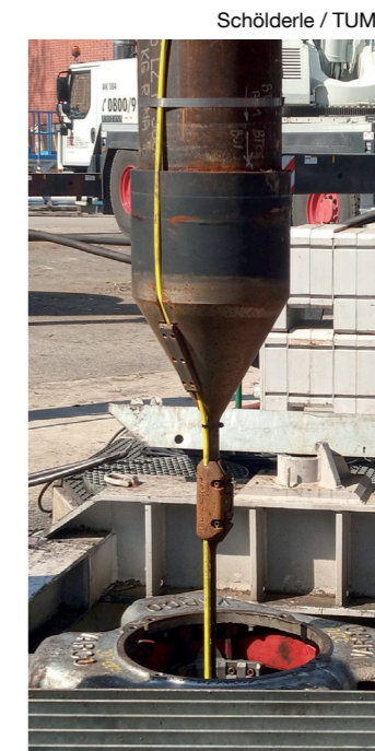
■ Fig. 1.: Installation of the fibre optic cable in a geothermal borehole.
