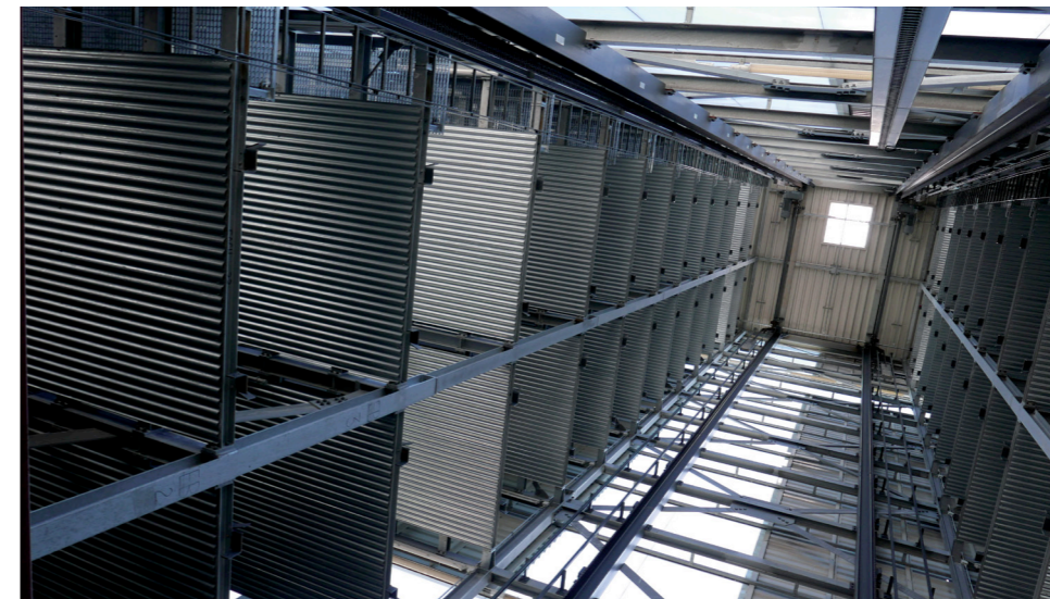
Fig. 4: Cartower with 12 levels for 2 cars each which could be converted to a Greentower with containers for vertical farming.
