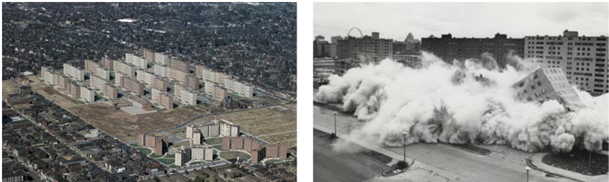
Figure 6-1: Aerial views of the Pruitt-Igoe complex before and after the explosion. Left: United States Geological Survey (public domain); right: U.S. Department of Housing and Urban Development (public domain)
