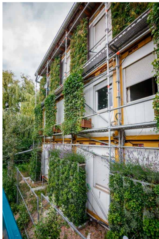
Figure 11. Three different systems of vertical greening were installed to investigate differences in performance. A scaffolding supports the plant boxes of the upper floors. Photo: Julian Rettig.
