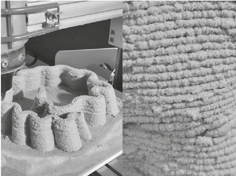
Figure 3. 3D print prototype with SC(left). Connection of printed layers of SC mortar (right) [Original from authors].
