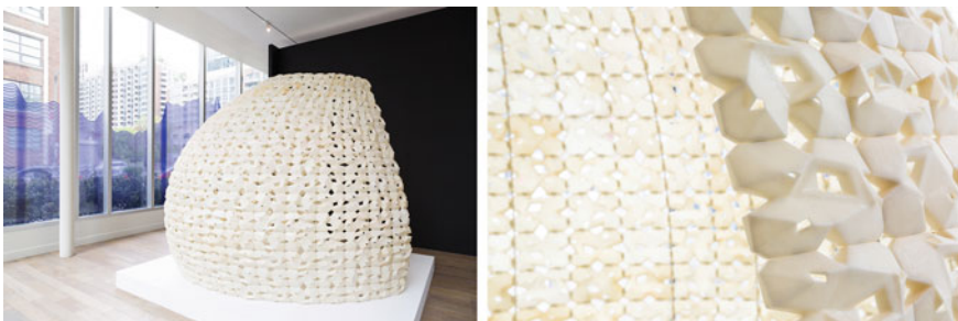
Fig. 4 Left and right—a 3D-printed salt pavilion. Source Emerging Objects/Ronald Rael and Virginia San Fratello [71]
