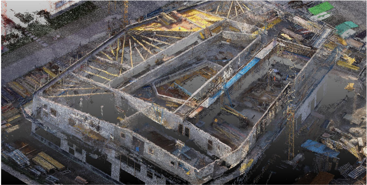
(a) Photogrammetric point cloud of construction site (Braun et al., 2020)
