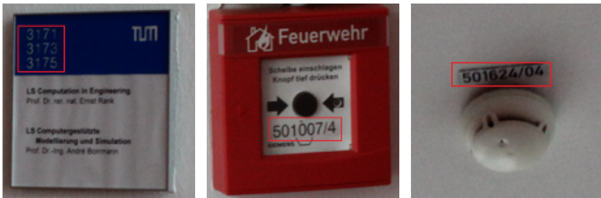
(a) Room number on door sign (b) Serial number on fire alarm switch (c) Serial number next to smoke alarm
