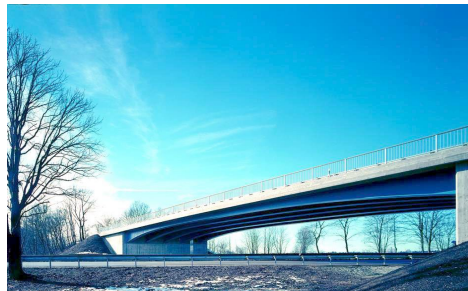
Figure 1. integral composite frame bridge
