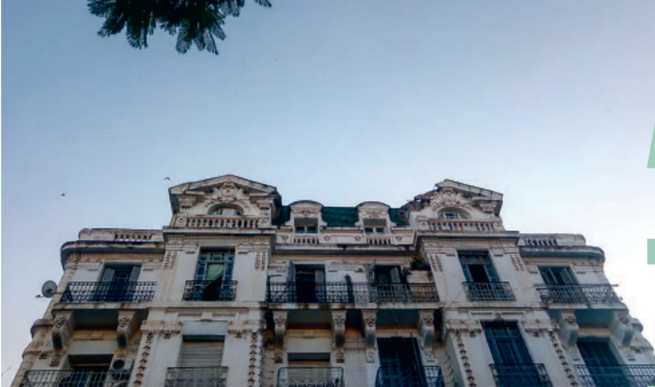
Fig. 2: An inhabited building which belonged to French settlers on Avenue of Paris, Tunis. Photo by Khaoula Stiti, 2018.
