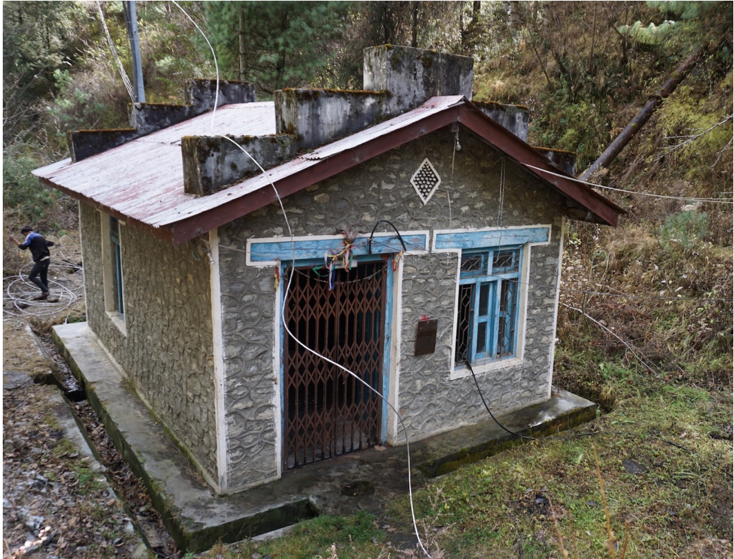
Figure 3.7: Chame power station and penstock [own illustration]
