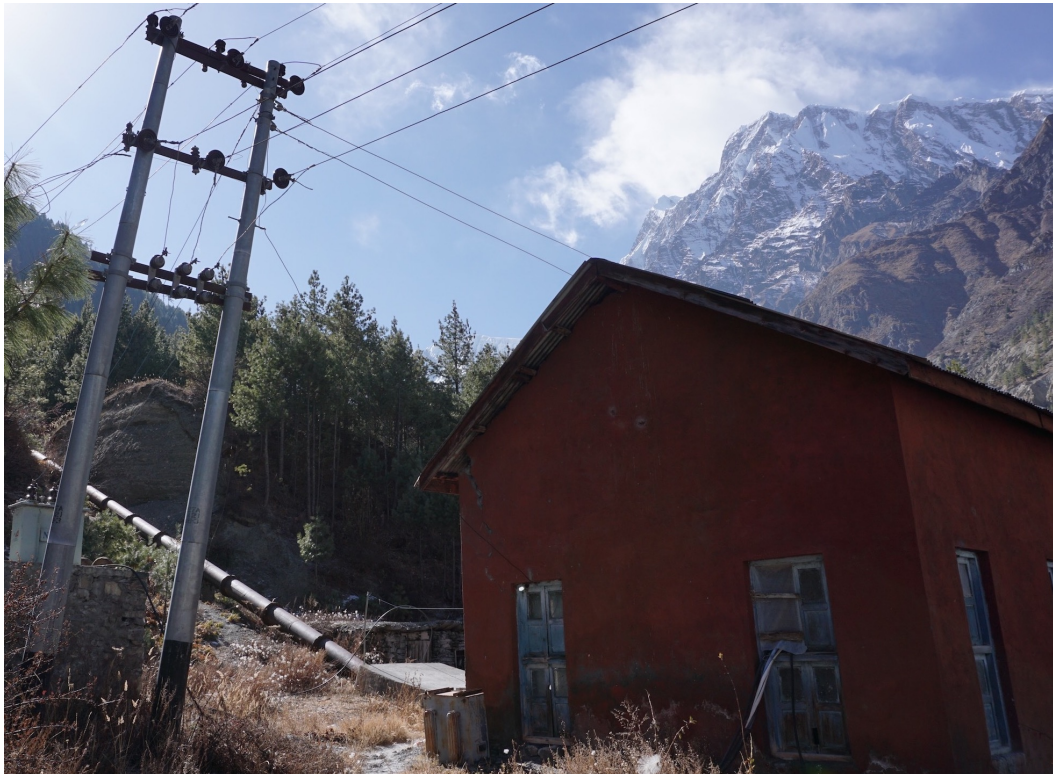
Figure 3.6: Sabje power station and penstock [own illustration]
