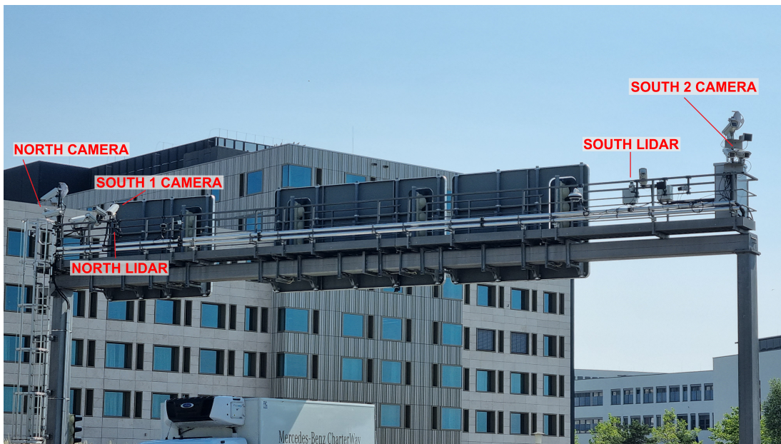
Figure 3.2: S110 gantry bridge with the locations of all of the sensors used in the TUMTraf Cooperative Dataset.
