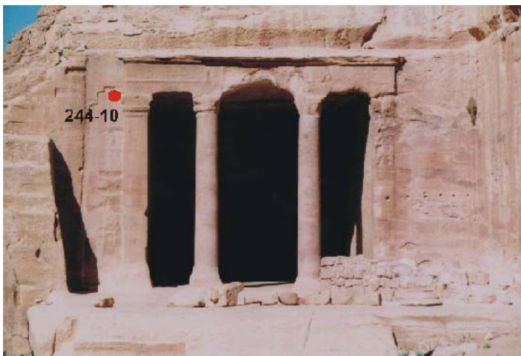
Figure 35. The Garden Temple (No. 244) with stucco remains in the form of ashlar masonry.
