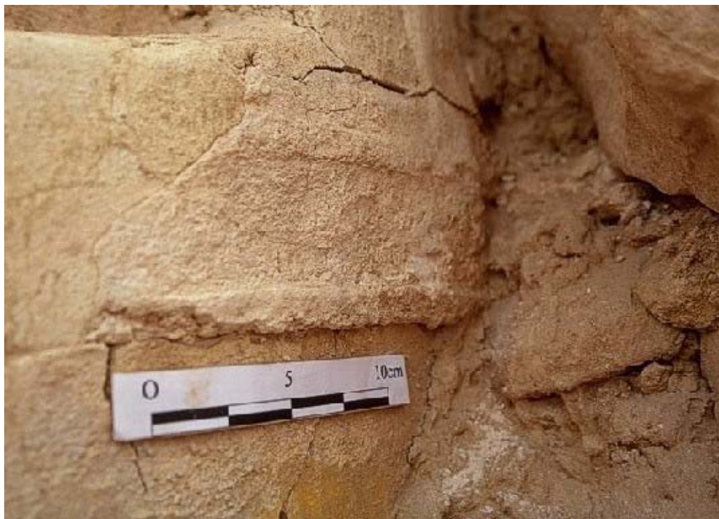
Figure 72. Moulded rim going around one of the columns, below which is a yellow painted and polished surface, while above it is white fluting.
