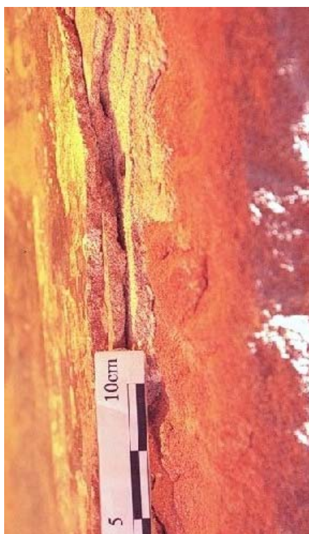
Figure 52. Lower part of wall: 3 layers.
