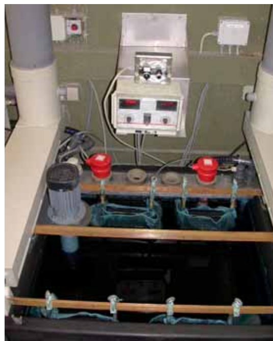
Figure 2.9. Image of electrolytic bath
