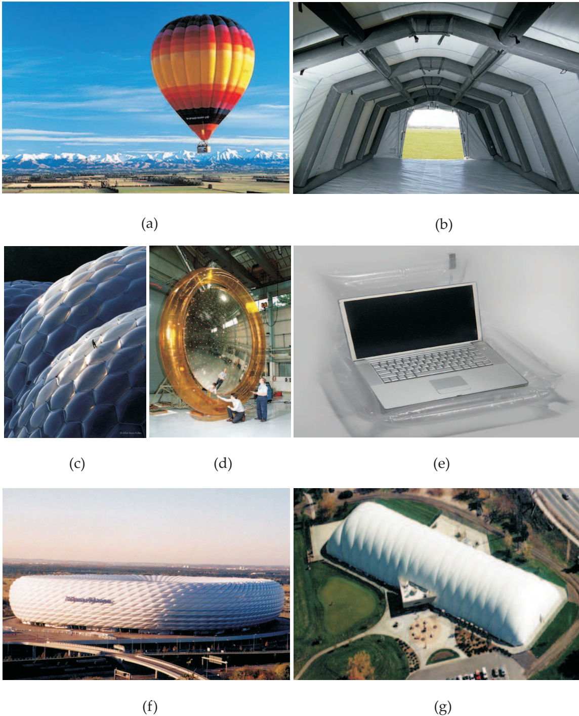
Figure 4.1: Applications of inflatable structures (a) hot air ballon ( http://images.google.de ) (b) rescue shelter supported by inflatable beams ( http://www.gumotex-rescue-systems.cz ) (c) pneumatic membrane roof for Eden Project, Cornwall, UK (d) space communication antenna with 6.4 m inflatable ring and 5 m inflatable reflector ( http://www.abc.net.au ) (e) inflatable packaging ( http://www.inflatablepackaging.com ) (f) air cushions cladding of the Allianz arena ( http://www.allianz-arena.de ) and (g) large span air house ( http://images.google.de )
